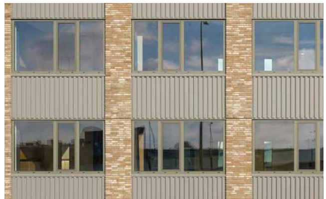
Project: Ruigrok Tower Aalsmeer › Montage: Total Cladding › Producten: SAB-Block 30/415 in Colorcoat HPS200 Ultra® Pure Grey
