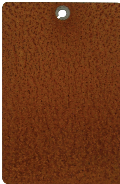
Mild steel corrosion coupon on freely exposed cladding showing lighter surface corrosion.
